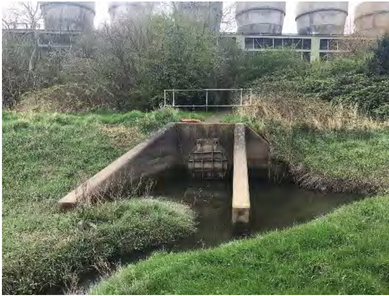
Plate 4: Outfall from culvert on Kelsterton Brook
