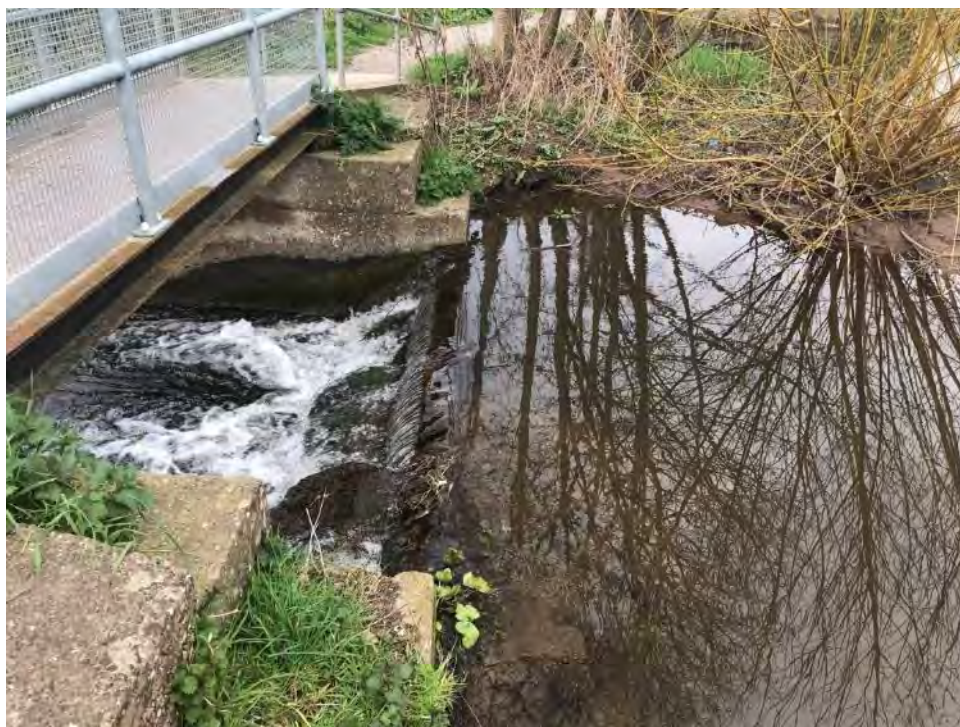
Plate 7: Weir on Pentre Brook
