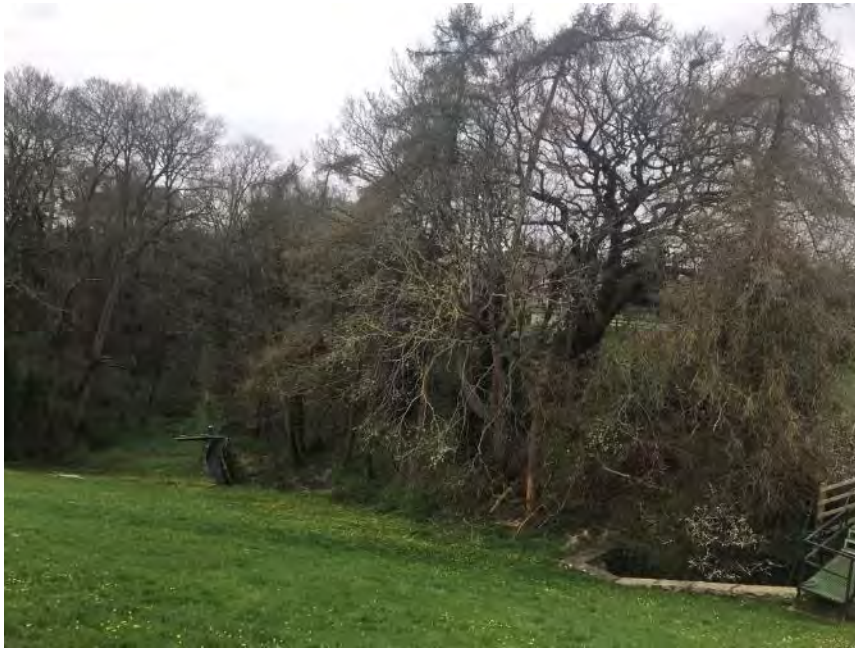
Plate 8: View to Lead Brook at bottom of spillway from reservoir
